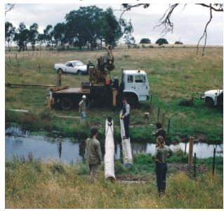
Old bridge pulled out, February 2022. Same view eastwards. Temporary embankments were created to contain the water coming into the reservoir prior to the concrete base being laid in March.
